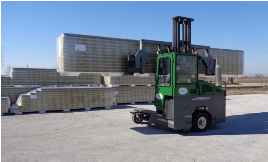
Pic 2. Unloading with forklift
