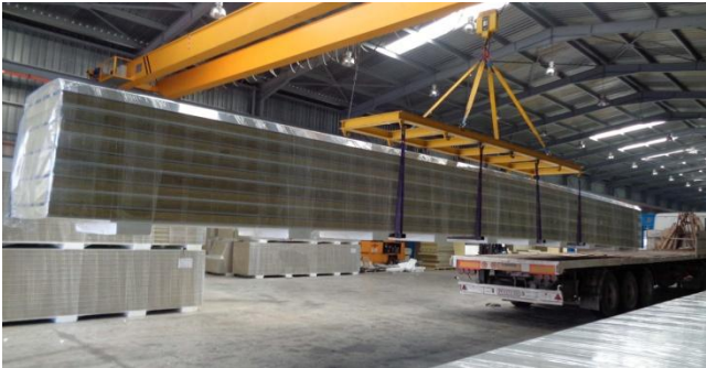
Pic 1. Unloading using crane and steel frame.
